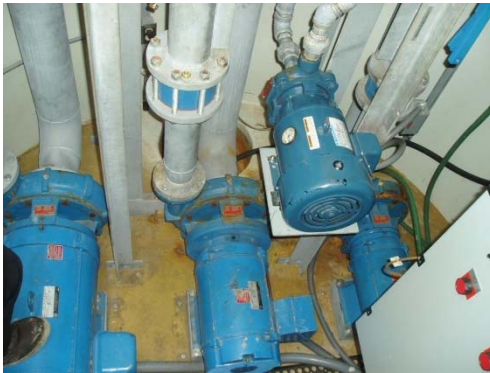
Exhibit 8 – Wortman Loop Pump Station
